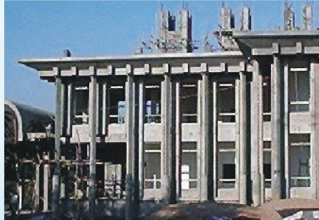
Long windows designed for Daylight Harvesting at Gulbarga
