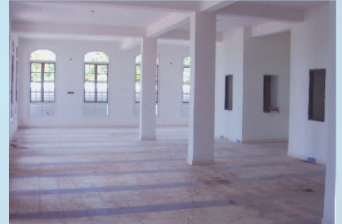
Long windows designed for Daylight Harvesting at Gulbarga
