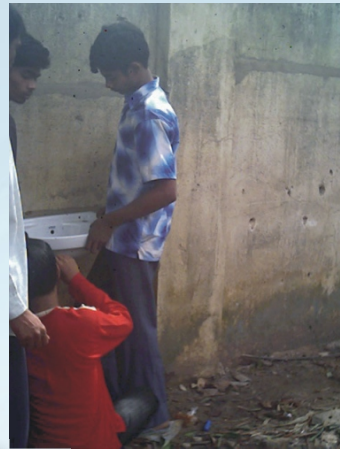
Fitting pipes to supply water
